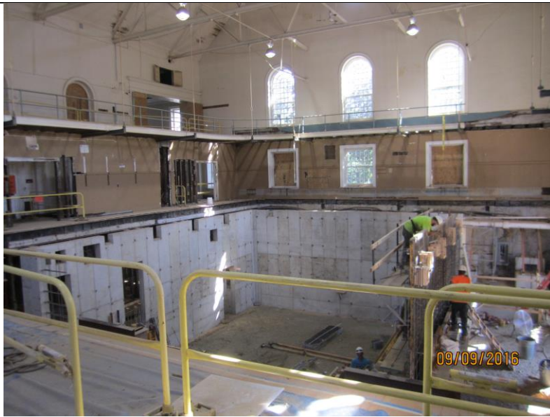
Left: Large opening in the gymnasium floor at the main floor diaphragm. Concrete shear walls were used to laterally re-support the existing structure.
