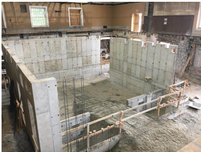
Left: Concrete shear walls laterally re-support the existing structure and provide the necessary acoustic requirements for the new performance space.
